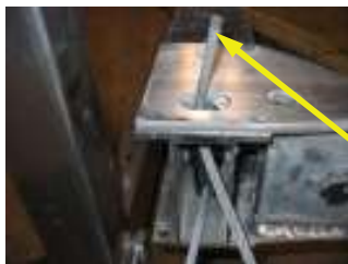
Winch column view of twin beam and front to back member together.
