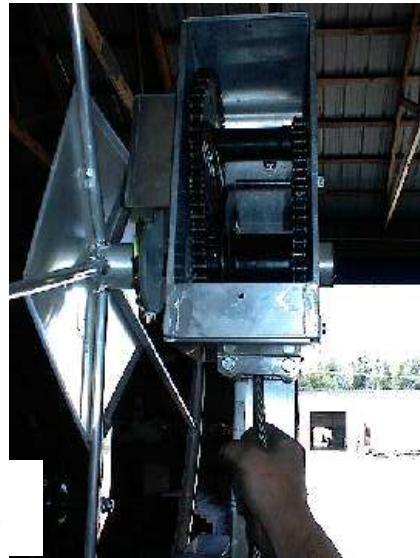
Then pull cable tight through bottom of winch.
