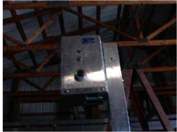
View of winch on column.
