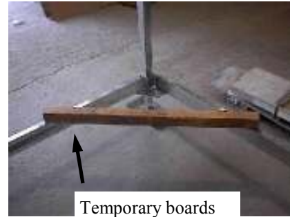
Another picture of diagonal use of the temporary boards.
