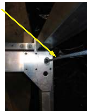
Non winch front of hoist corner. Parts are fit together.
