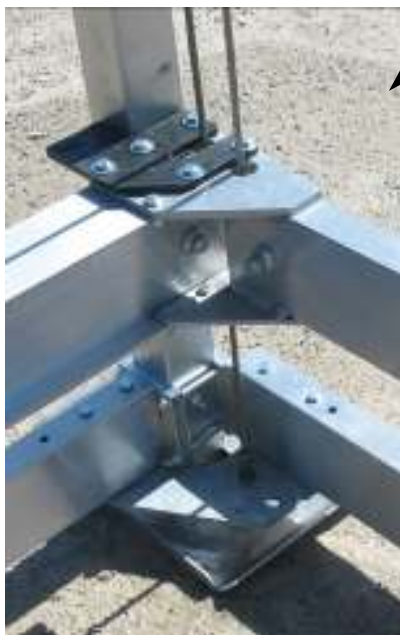
Rear Column area assembled
